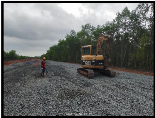
Crushed Stone Laying Work
