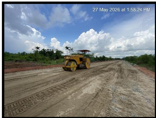
Crushed Stone Compaction Work
