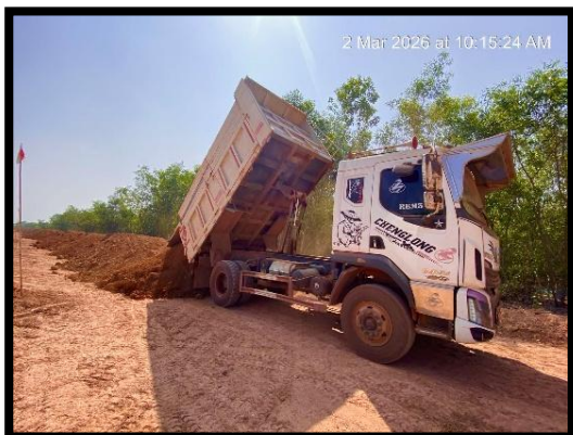
Borrow Soil Laying Work
