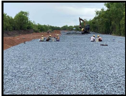
Crushed Stone Laying Work
