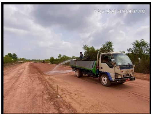
Soil Compaction Work
