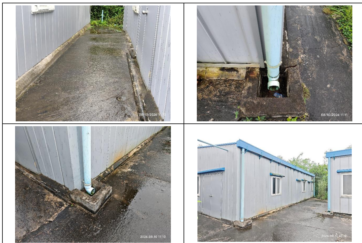
Figure 4-4 Storm Water and Drainage System at Project Office
