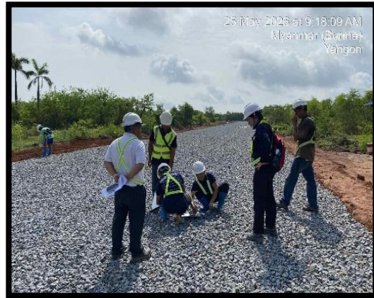
Crushed Stone Moisture Content Test
