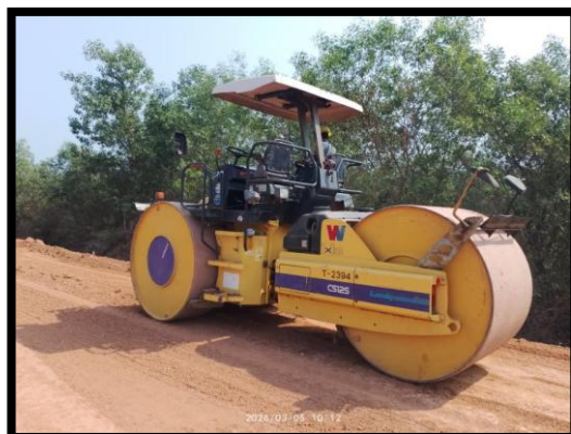
Soil Compaction Work
