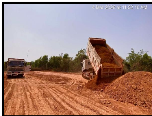
Borrow Soil Laying Work
