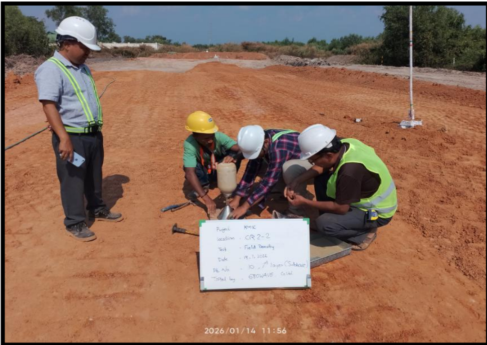
Item : Field Density Test Description : CR2-2 Date Taken : January 14, 2026
