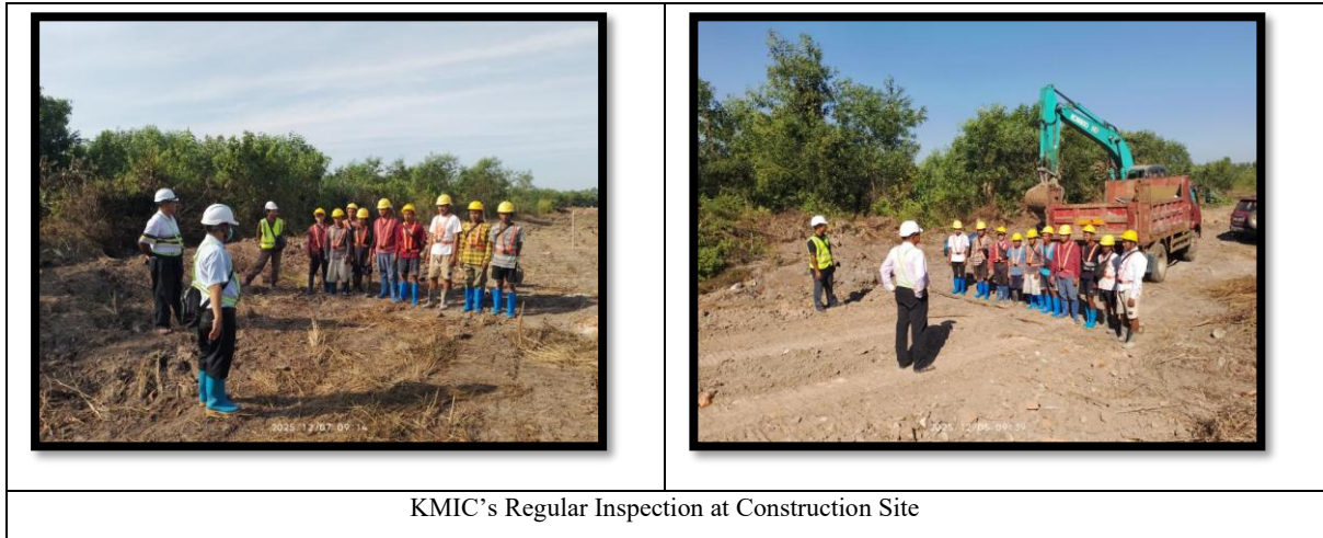
Figure 5-1 On Site Checking and Site Inspection
