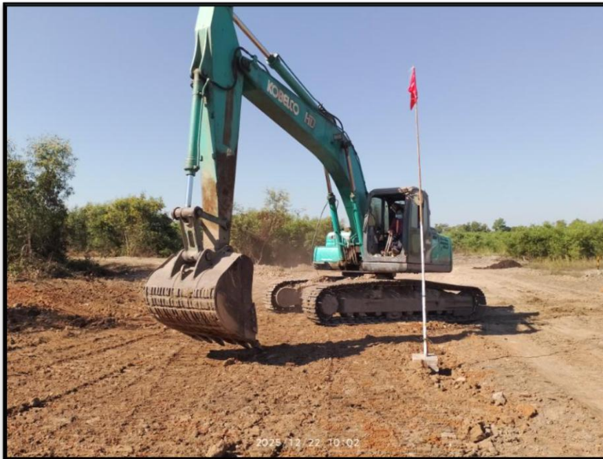
Item : Earth Work Description : Access Road Preparation work Date Taken : December 22, 2025
