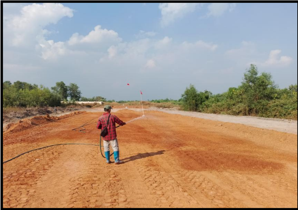
Item : watering work Description : CR2-2 Date Taken : January 14, 2026
