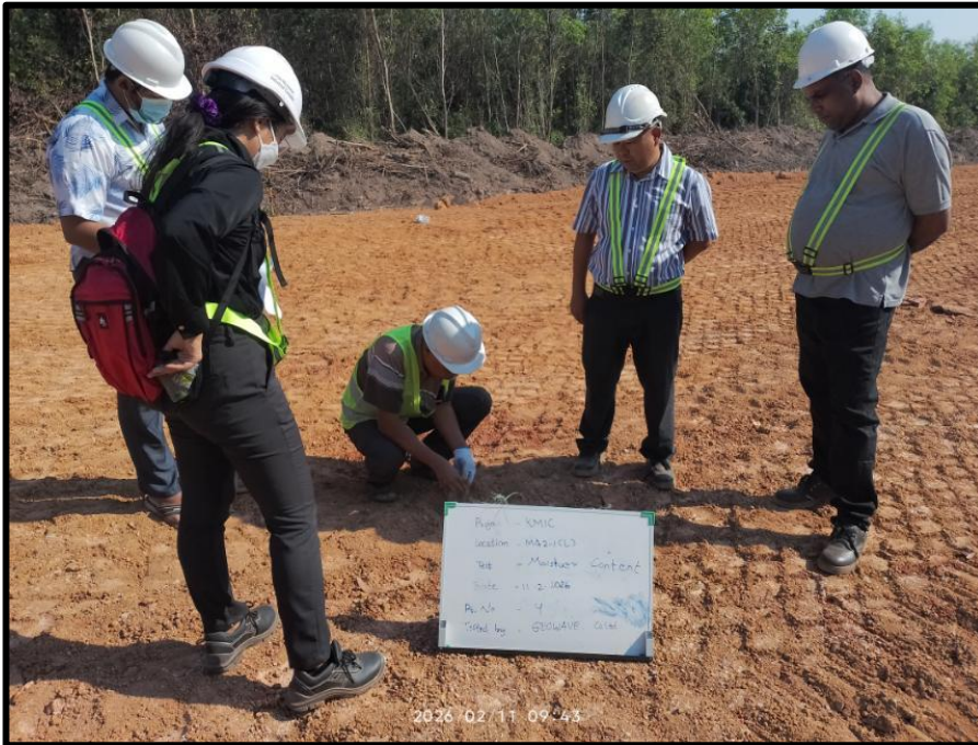
Item : Moisture Content Test Description : CR2-16,CR2-2,MA2-1(L) Date Taken : February 11, 2026
