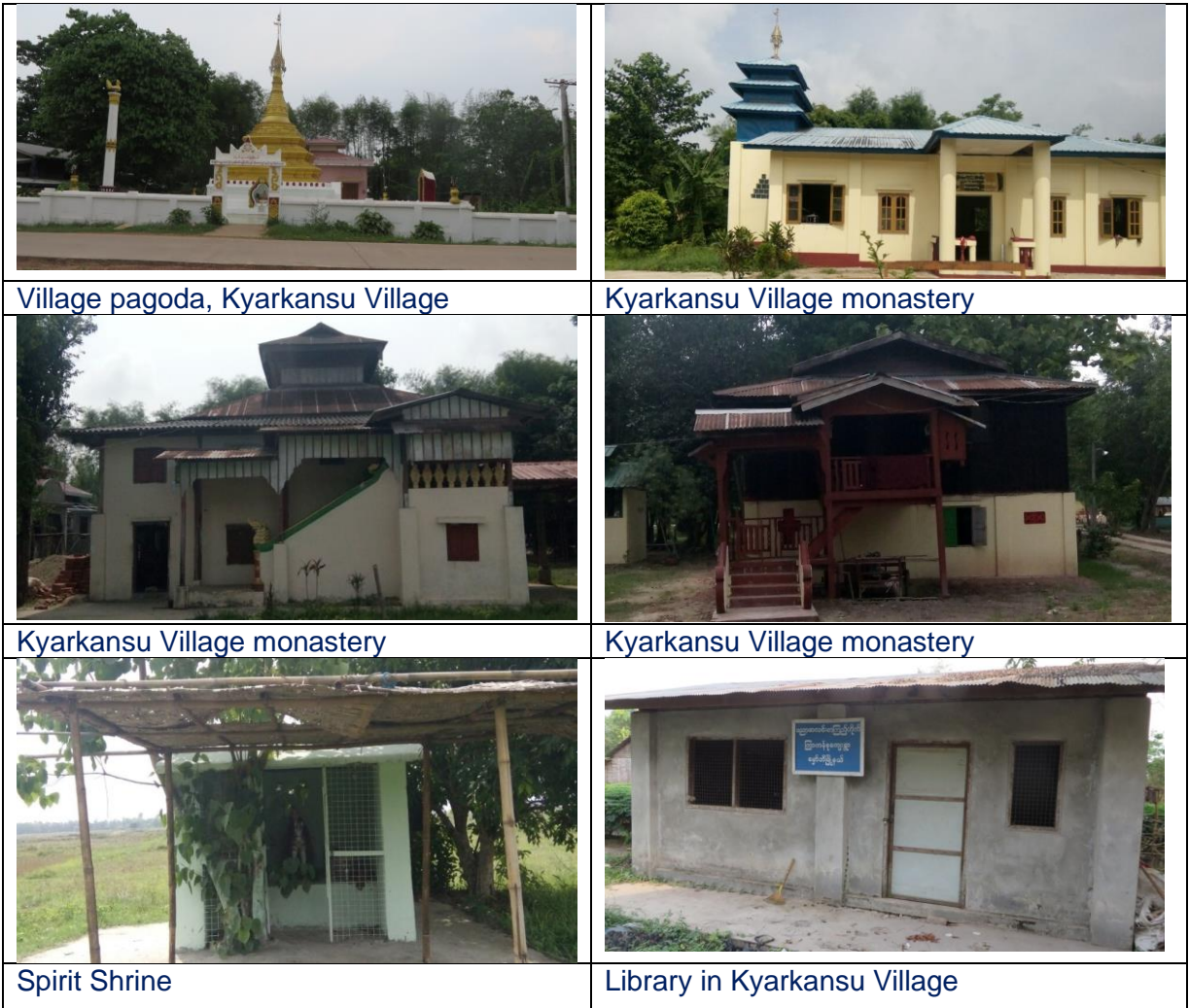
Figure 4. 70: Kyarkansu Village Buildings
