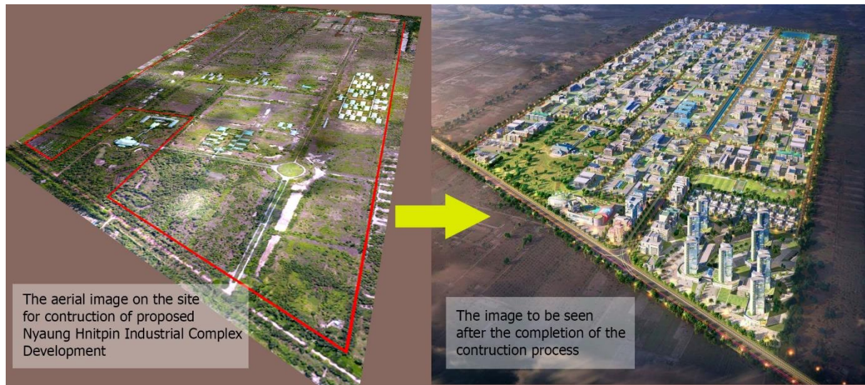
Figure 3. 1: Overview Image of Project
